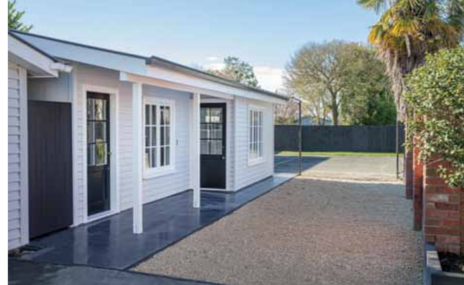
LEFT The pool house is flanked by Boston Black Honed Granite tiles from Stone and Tile Solutions.
